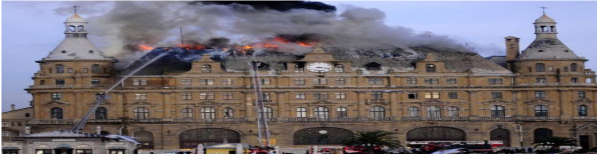
Figure 1. Haydarpaşa Train Station Fire (Özgünler, 2018)
