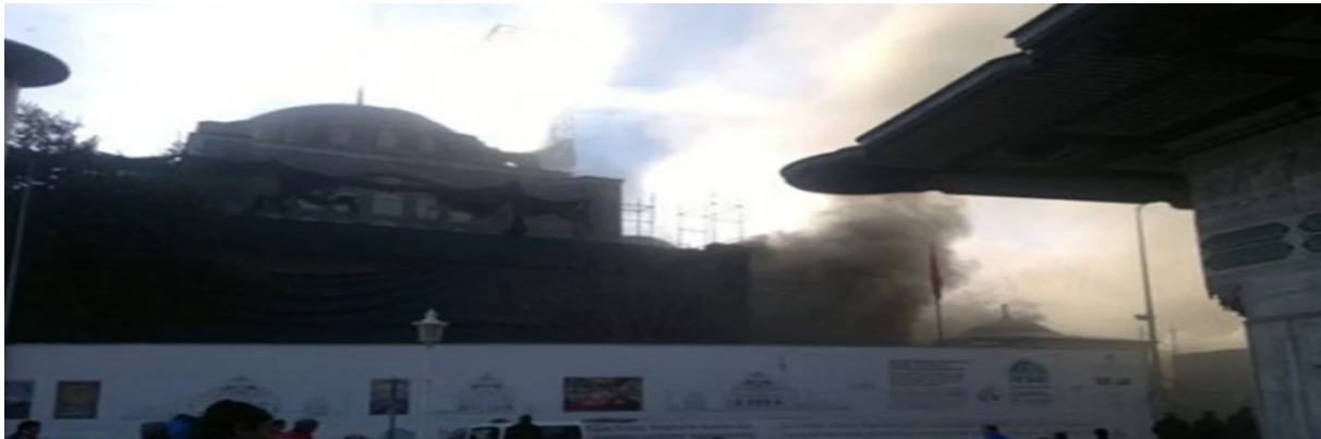
Figure 2. Kılıç Ali Paşa Mosque Fire (URL 2)
