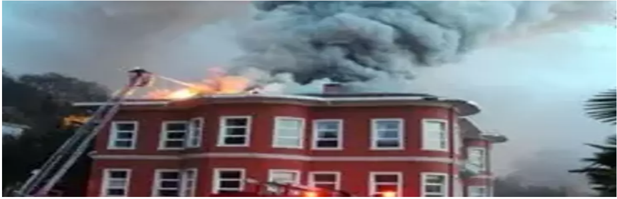
Figure 7. Müşir Fuat Paşa Mansion Fire (Yalçın, 2013)
