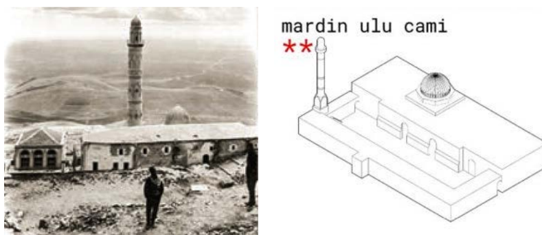
Picture 13. The hipped roof of the Mardin Great Mosque in 1911 (Gertrude Bell Archive) (left) Figure 7. Today's flat roof (URL 4) (right)
