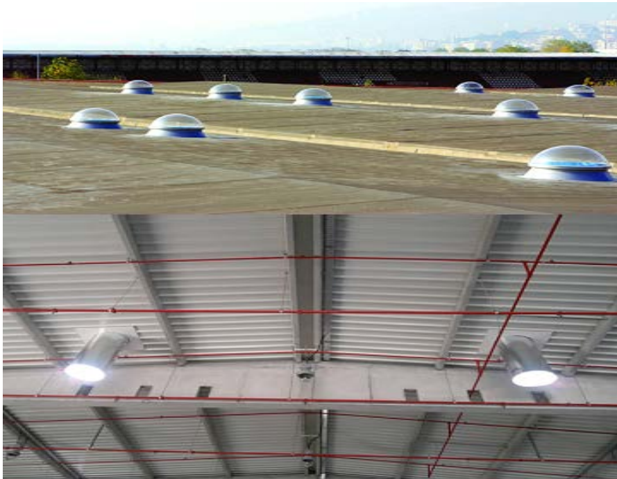
Fig. 5. Bottom and roof top view of the light tube for a warehouse
