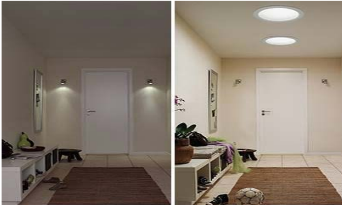
Fig. 4. Reflection of daylight by the diffuser before and after light tube application
